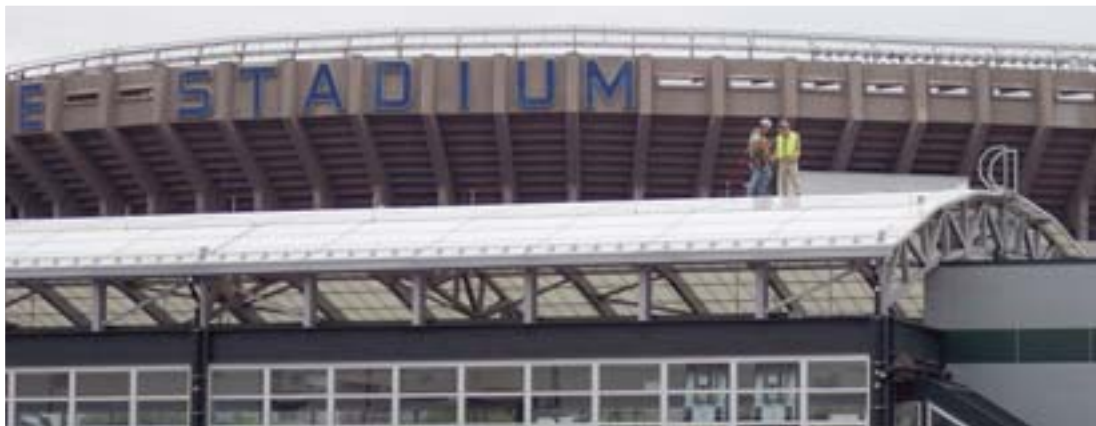
Atop the rail station, workers can safely walk across the skylight.
