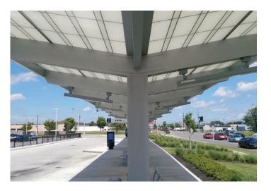
The center includes an 8,950-square-foot overhead canopy system that integrates a single-source, aluminum box beam superstructure designed by Structures Unlimited, Inc. and featuring Kalwall®
